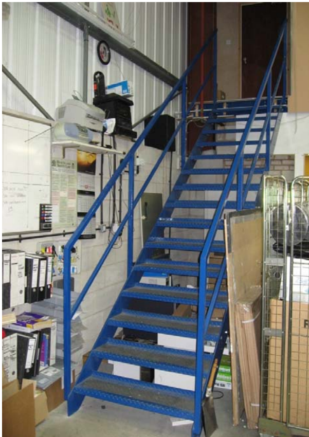
Four examples of different types of RDA Part K staircases – With open back risers, durbar steel plate treads, fully welded RHS handrails or RHS posts with galvanized steel tube handrails
